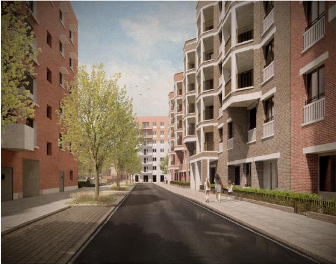
A view south along Alvey Street towards plot 4D.
