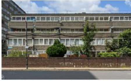
1. A view north from Kinglake Street to the existing buildings
